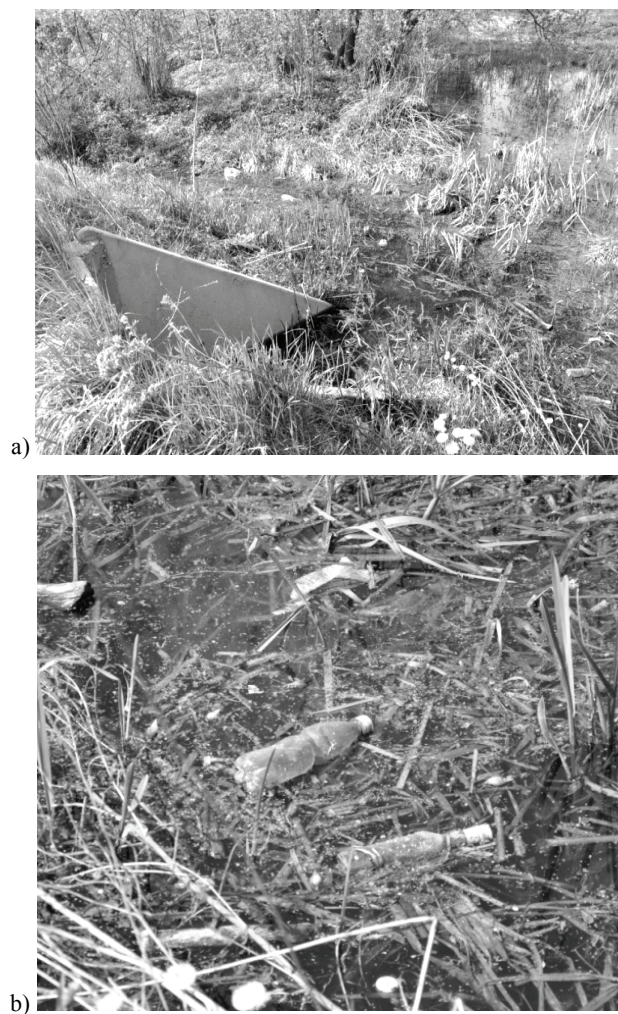
Fig. 3. a) connection of the Zemborzycki Reservoir and the studied water reservoir with a concrete sluice, b) present development and usage status of the water reservoir
