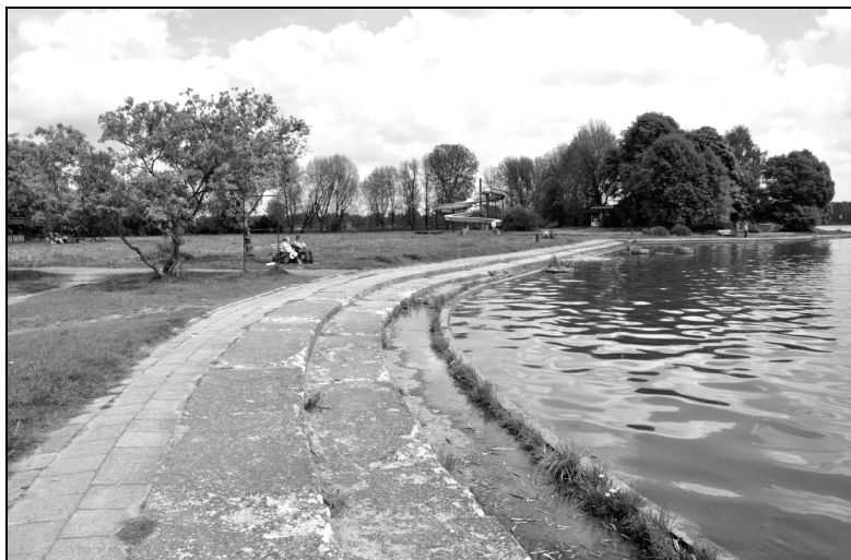
Photo 1. The concrete-strengthened western bank of the Zemborzycki Reservoir (Kułak 2009)
