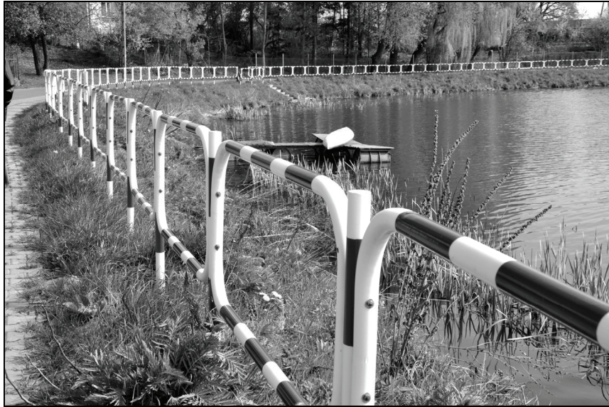
Photo 3. Railing along the bike path on the Zemborzycki Reservoir (Kułak 2010)
