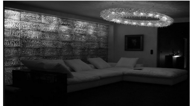
Fig. 5. Wall made of the translucent concrete Litracon [21]
