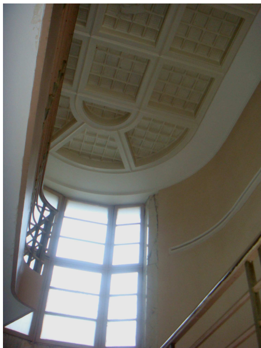
Phot. 22. The painted authentic glass blocks on the ceiling of the stairs hall of the Kassler building in Lviv
