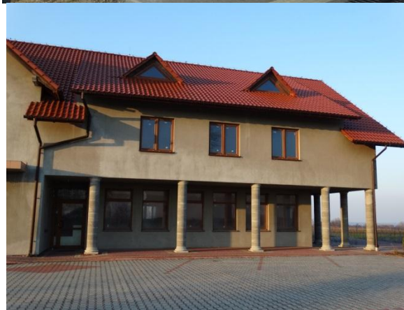
Fig. 2. Buildings with overhang without pillars and overhang supported by pillars (Foto: M. Buško)
